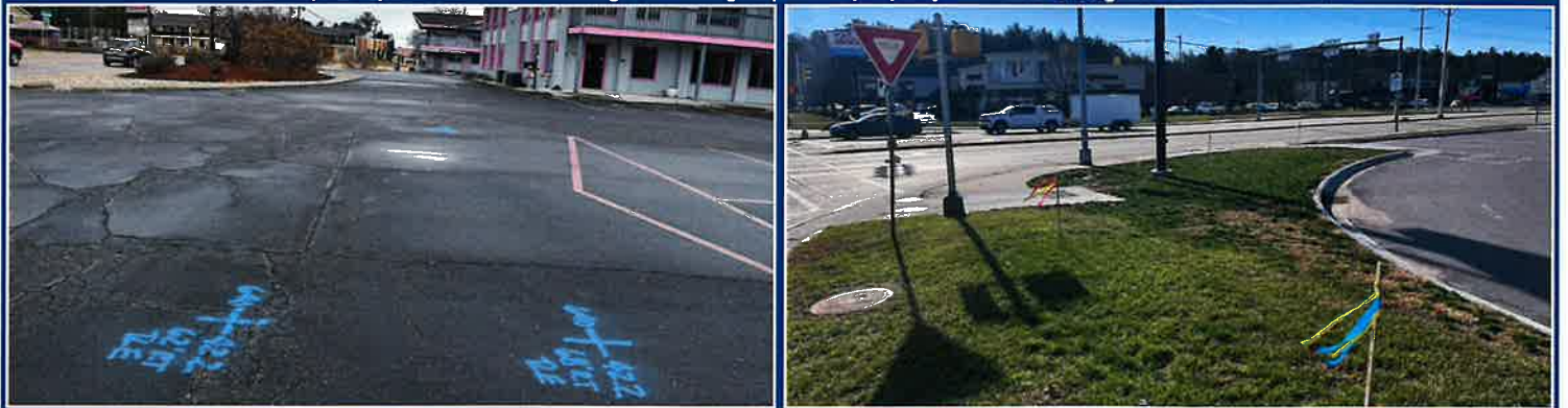
Example of paint and lath markings showing impacted property locations along the US 12 corridor.
